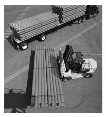
PVC and CPVC are strong, lightweight materials, about one fifth the weight of steel or cast iron. Piping made of this material is easily handled and, as a result, there is a tendency for them to be thrown about on the jobsite. Care should be taken in handling and storage to prevent damage to the pipe.
